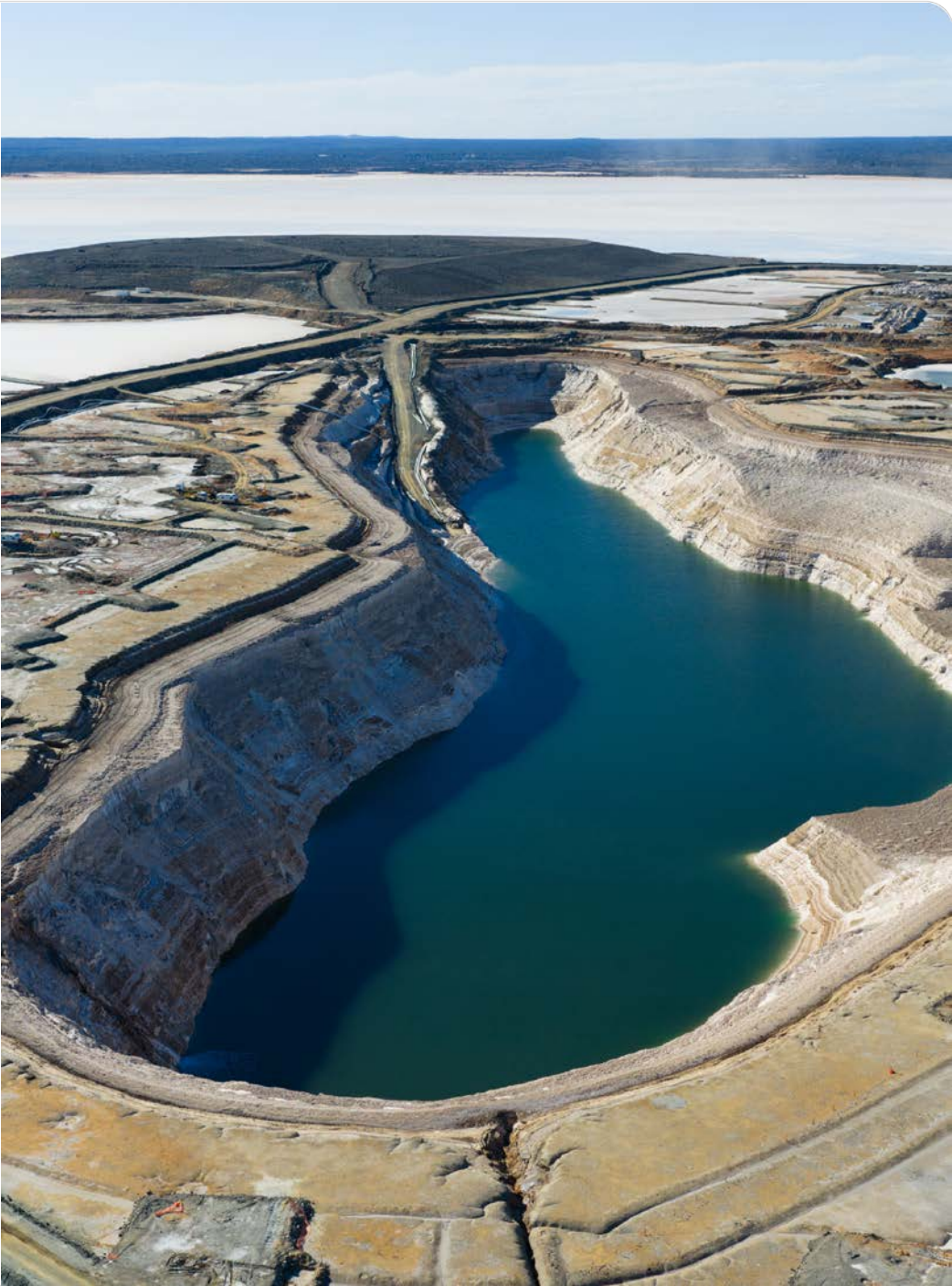
St Ives tailings facility
